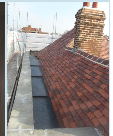
The refurbished roof
