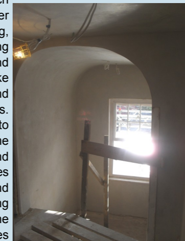
Lime plastering to the stairwell
